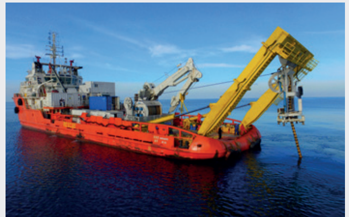
Subsea cable installation
