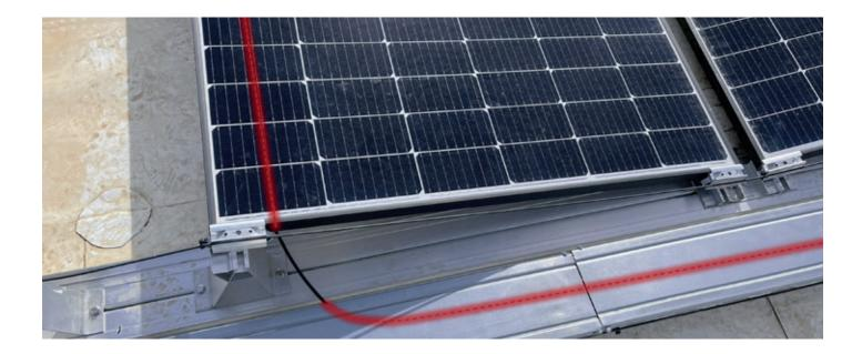
approximately 3.6 km, all in a single-ended configuration. The fiber optic cable zigzags between each row of solar panels in order to continuously measure the temperature of both the solar panels and the roof in case a fire were to develop below the roof or in a cable tray.
