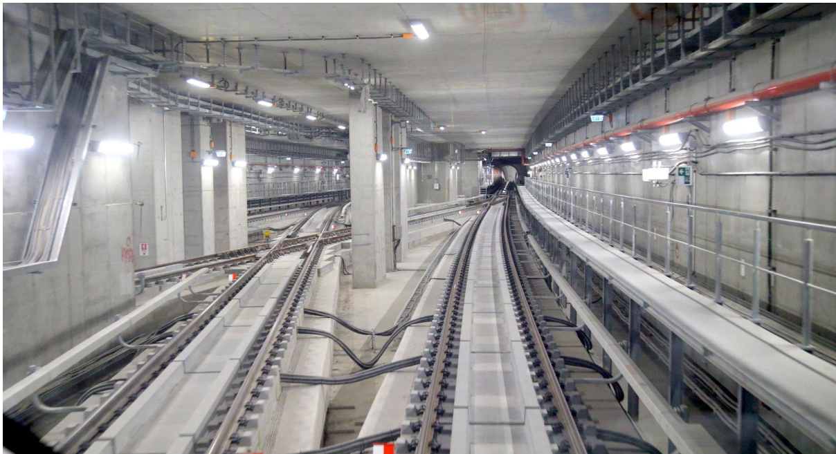
Tunnel along the Doha Metro line
