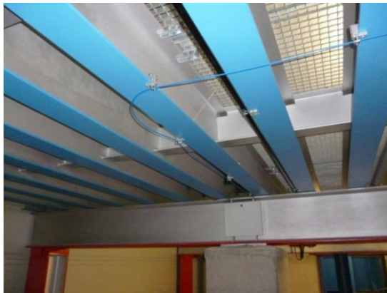
Sensor fiber installed along the production line route
