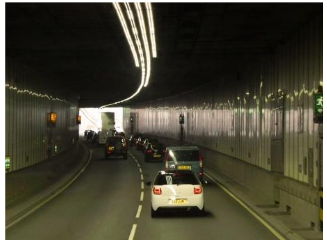
Meir tunnel: open for safe traffic
