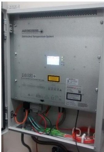
DTS wall unit fully installed
