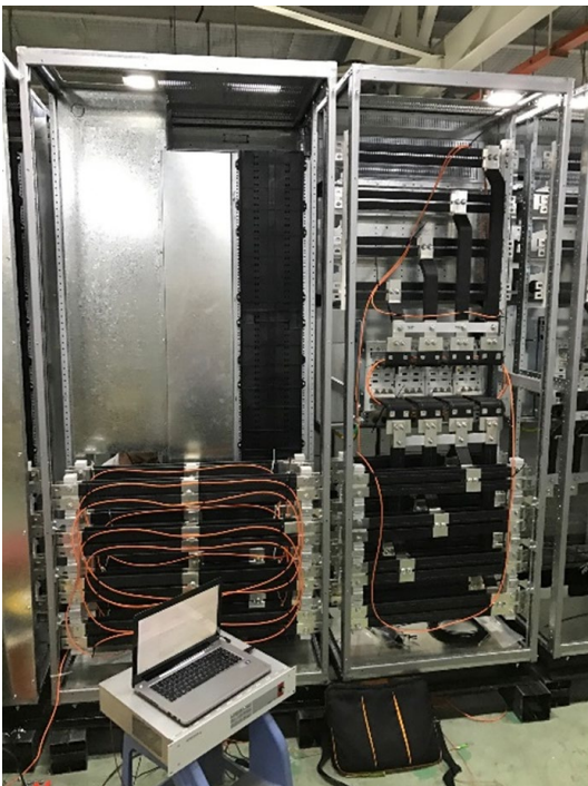
Testing the cable installation onto busbar of low-voltage switchgear
