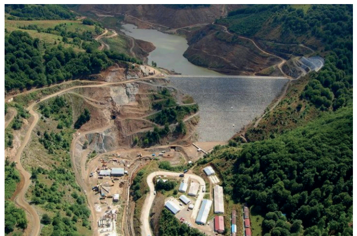
Figure 2: Knezevo Dam overview
