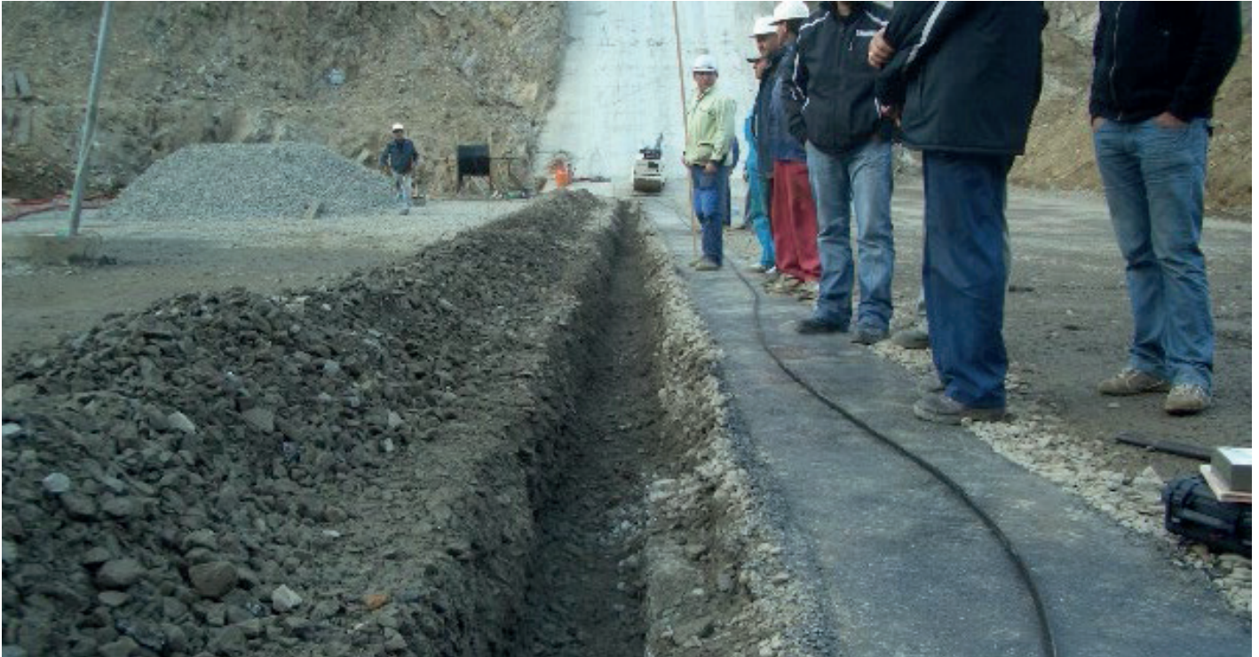
Figure 1: Cable installation
