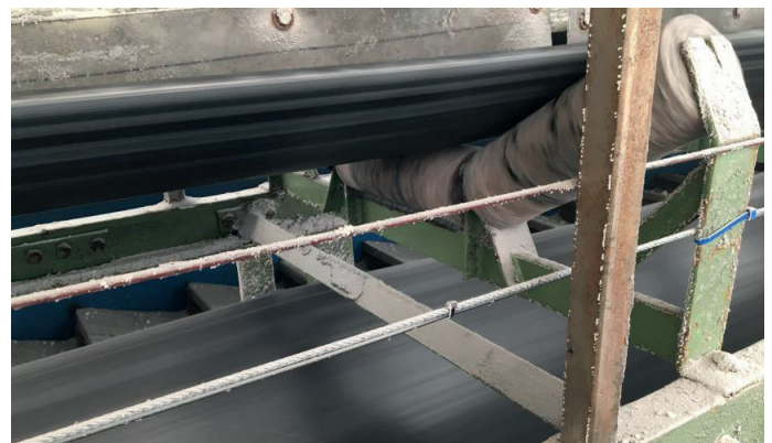
Figure 2: Cable installation (black), attached to the tension wire
