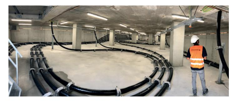
temperature information for all phases of the buried 220 kV and 380 kV power cables. With this 24/7 real time monitoring data, the operator is able to maximize circuit utilization and prevent failure in emergency situations.
