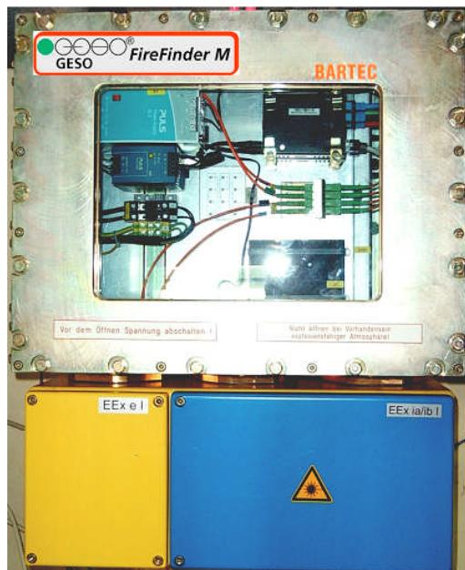
Fig. 8 GESO measuring station in pressure resistant enclosure
