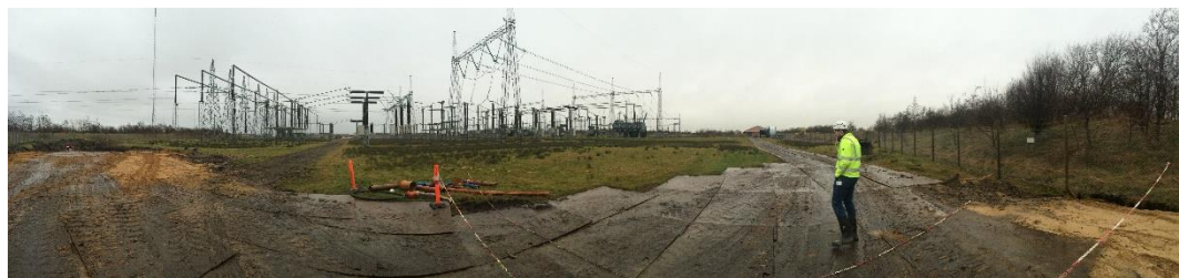
Underground cable route inspection
