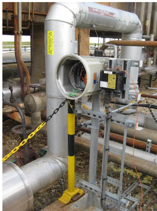
The remote end of the sulfur pipeline
