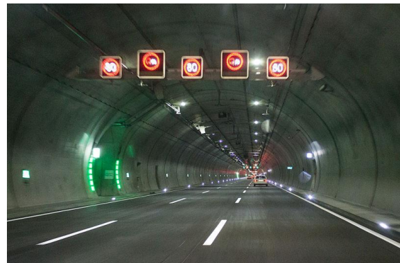
Northbound tunnel shortly before opening
