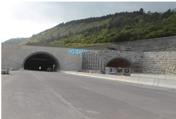
Jagdberg tunnel: Early construction phase
