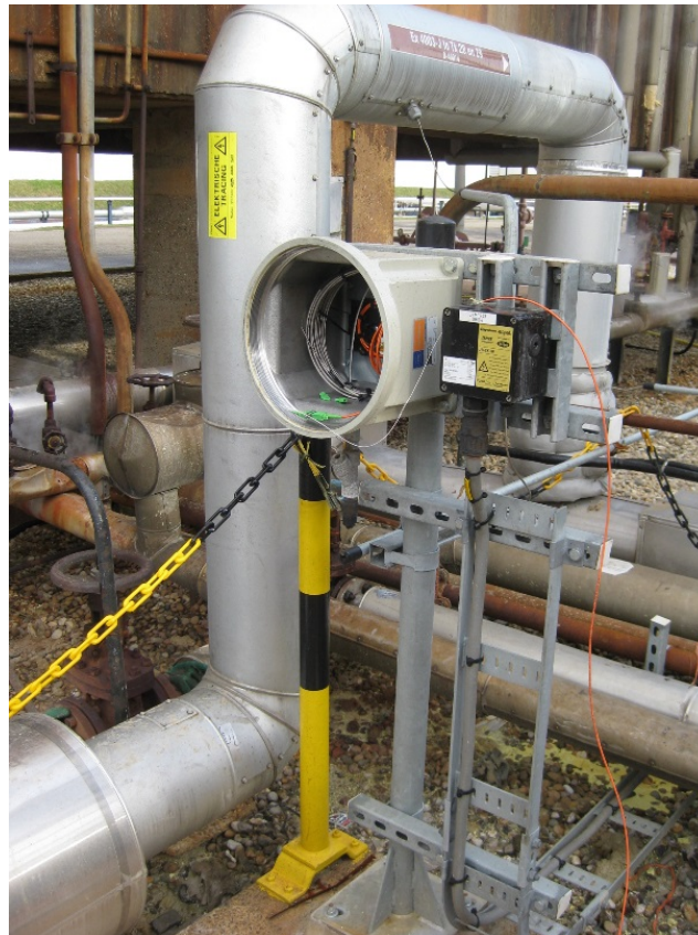
The remote end of the sulfur pipeline
