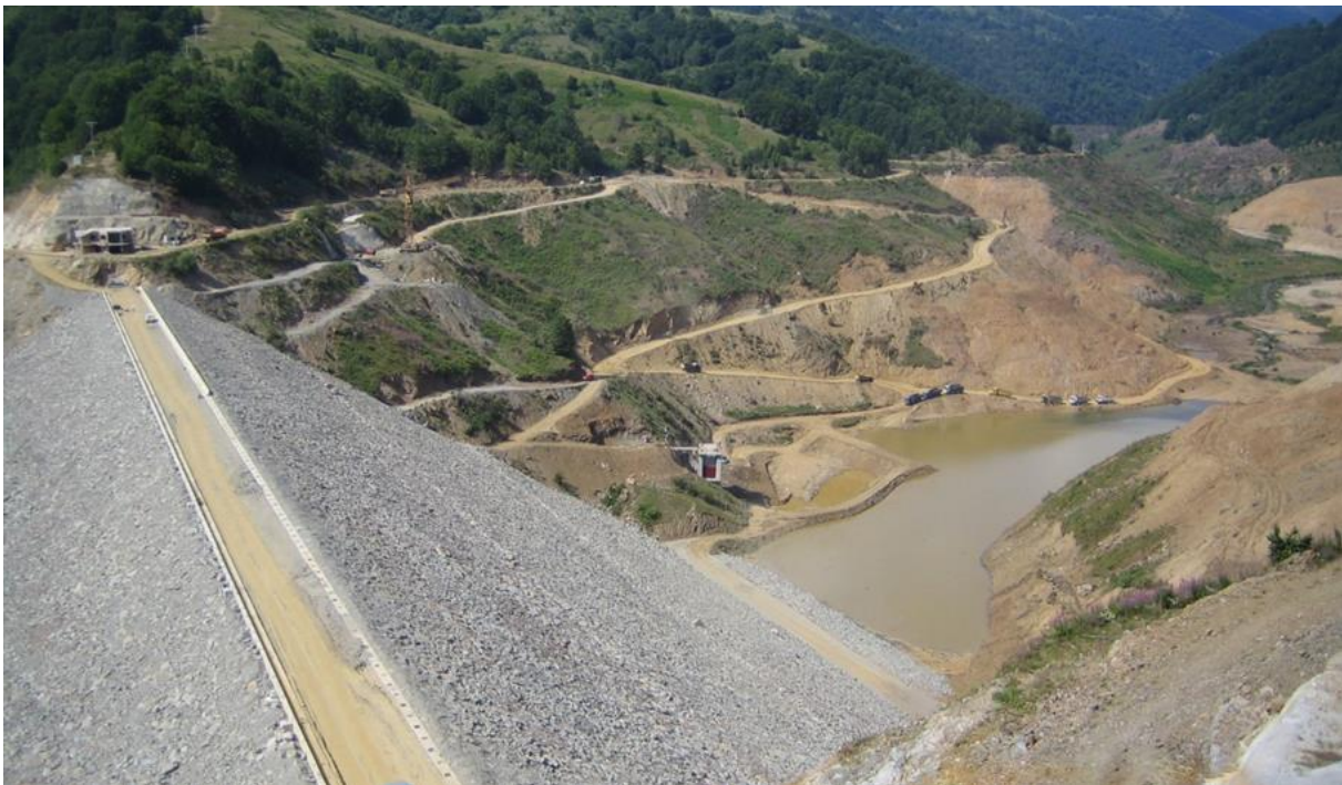
Knezevo Dam: late construction phase
