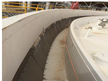
Fig: FO Cable mounting on Rim seal area of a FRT.
